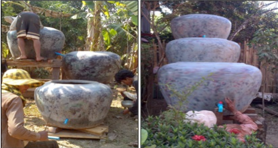
Figure 2: An angled 3-tier system being constructed in Kachon village (Left), and a straight 3-tier system in Vuen Sai Village (Right).
