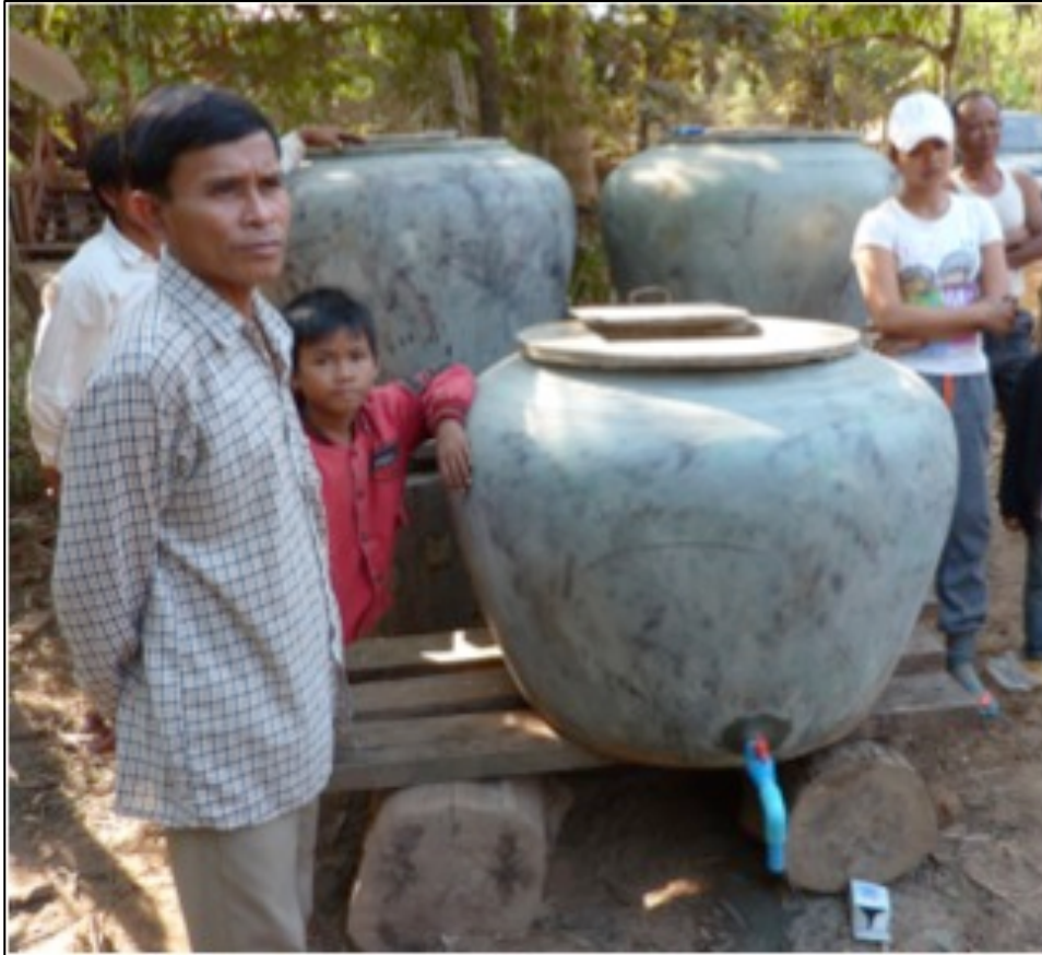
Figure 4: Ban Pong Village Chief (Left) and Ban Pong SEM Group Leader (Right) beside their water treatment system with an un-raised settling tank.
