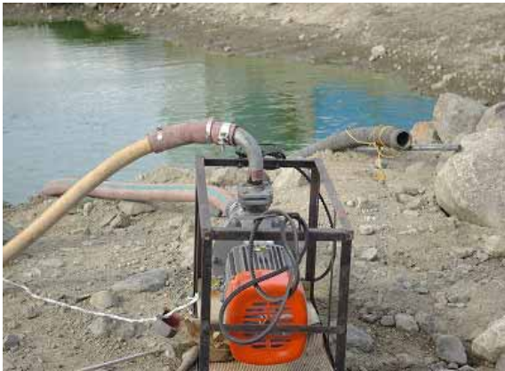
Pump at the temporary reservoir
