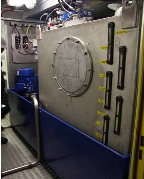
Oil tank for the hydraulic jacks in the foundation
