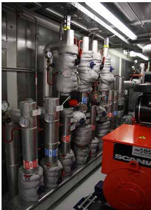
Water heating pipes using the exhaust heat from the generators
