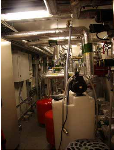
Generator heat exchanger
