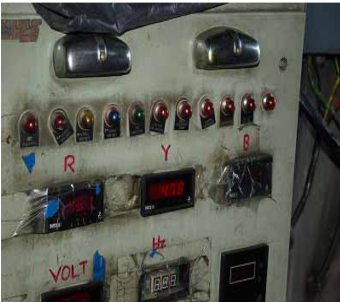
The monitoring panel of the power generator
