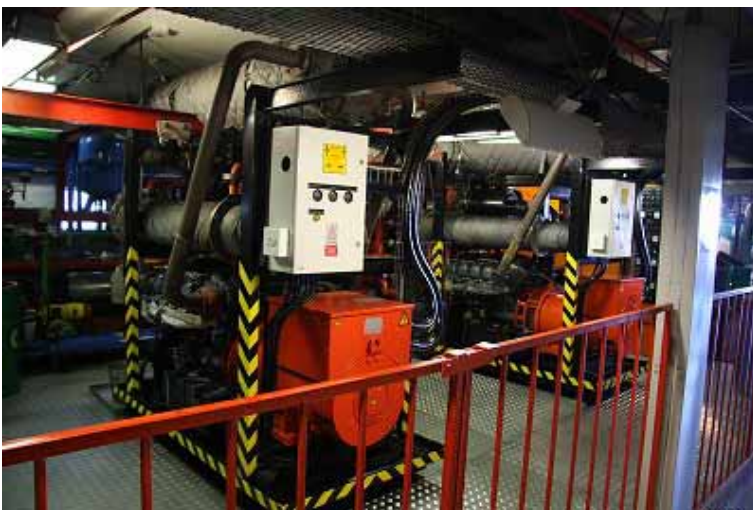
Diesel power generators
