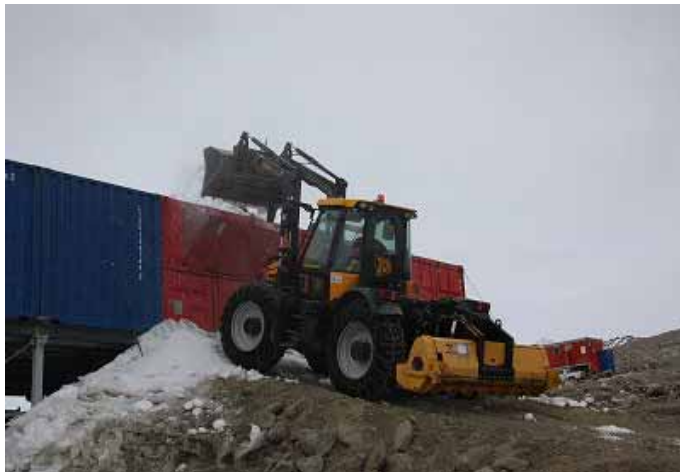
Putting snow into the snow melting system
