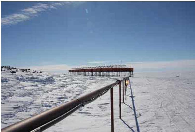
Oil supply pipes
