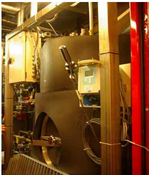
Sewage treatment tank
