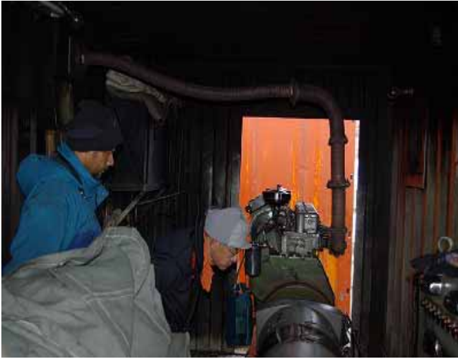
Air-cooled power generator
