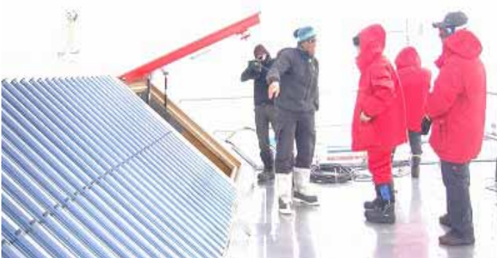
Solar panel for water heating
