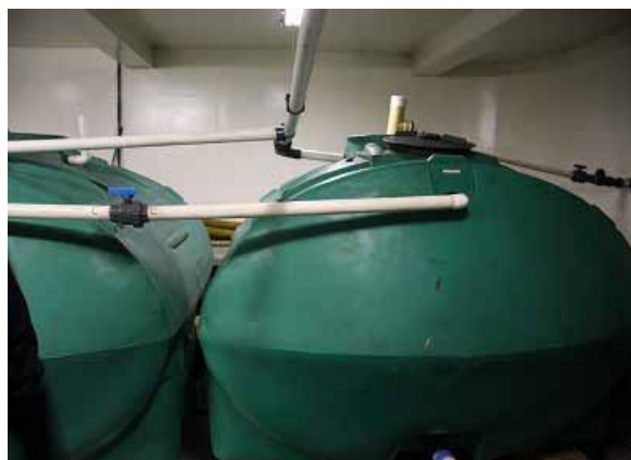
Sewage treatment tank
