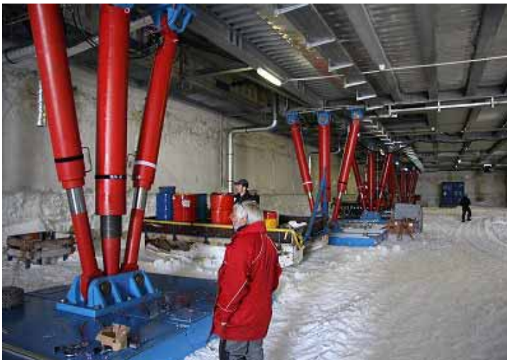
Supporting legs of the foundation of the station
