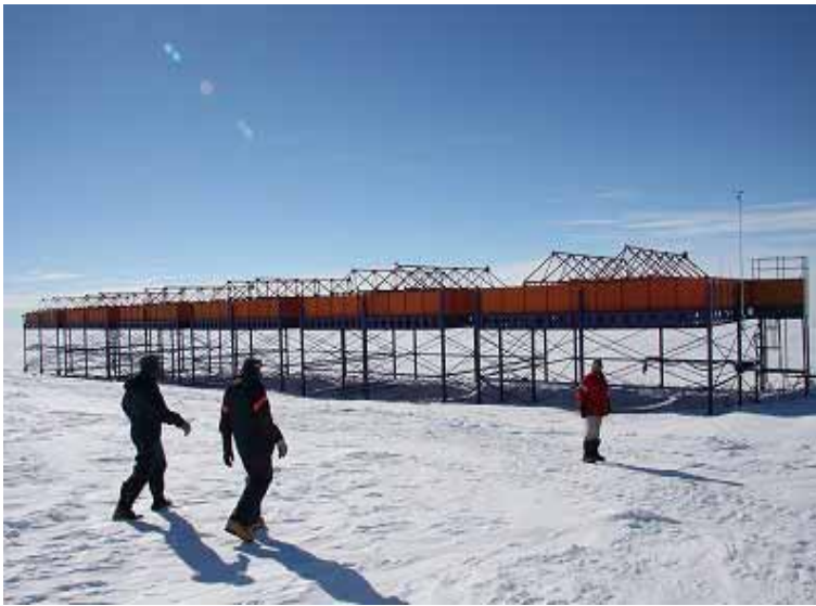
Oil storage tanks
