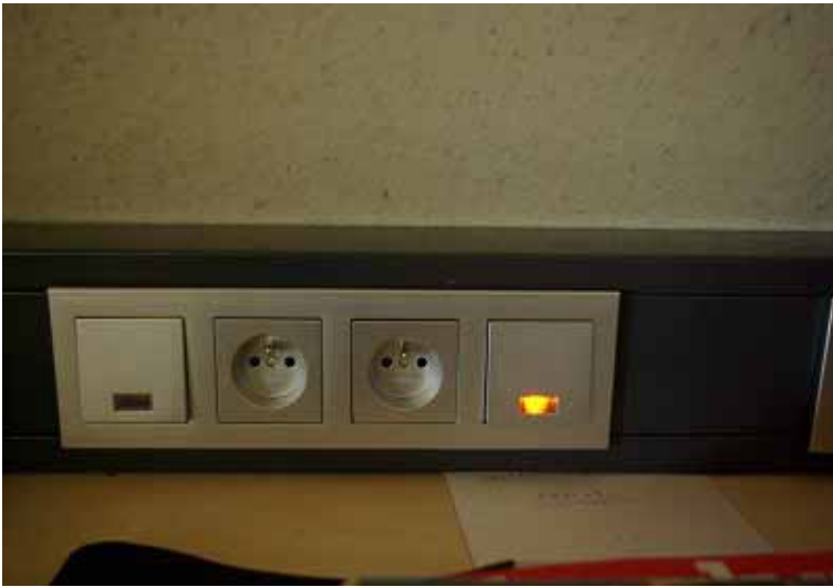
Outlets controlled by the smart grid (When energy is available, the light turns on after pressing the outlet button)
