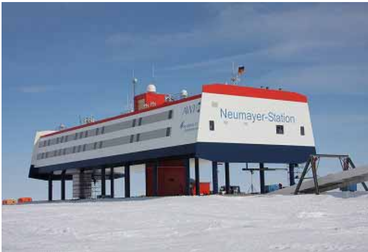
Exterior view of the station
