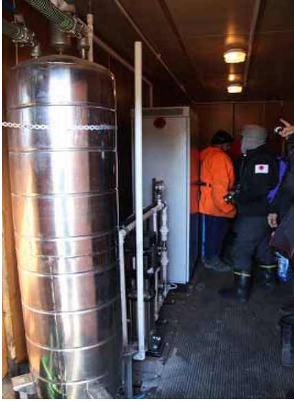
Ozone treatment unit for sewage water
