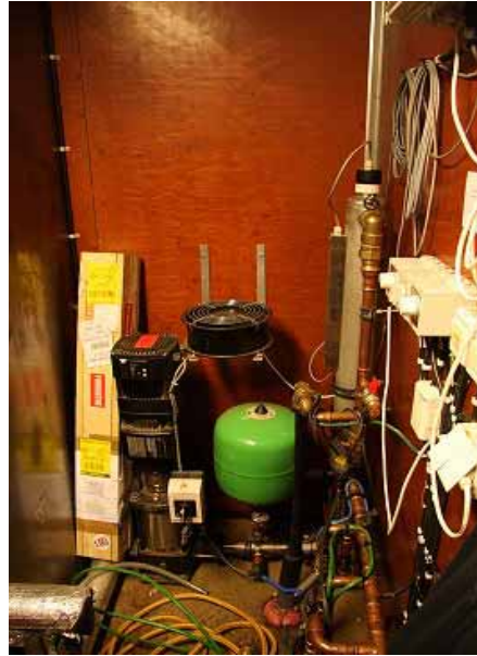
Water purification equipment
