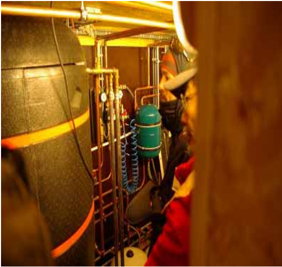
Hot-water tank and pump for making water
