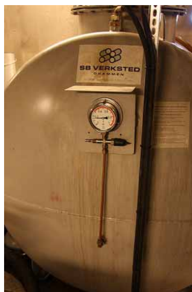
Fuel tank for generators
