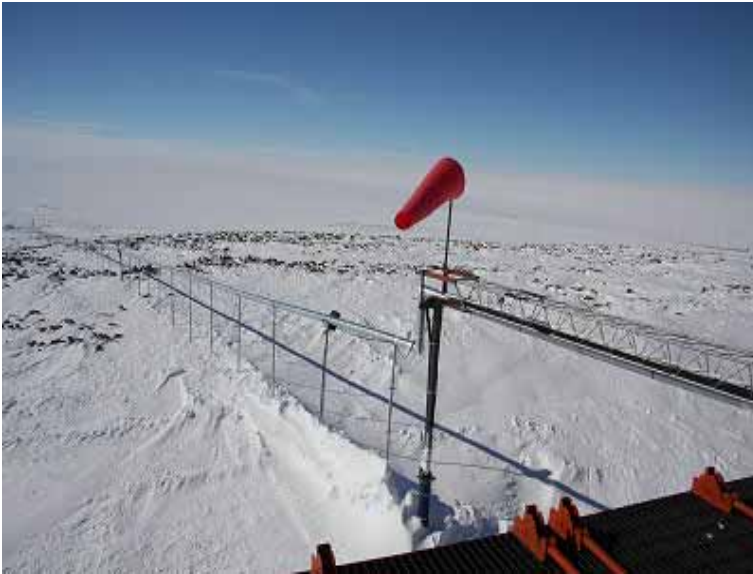
Water intake pipe
