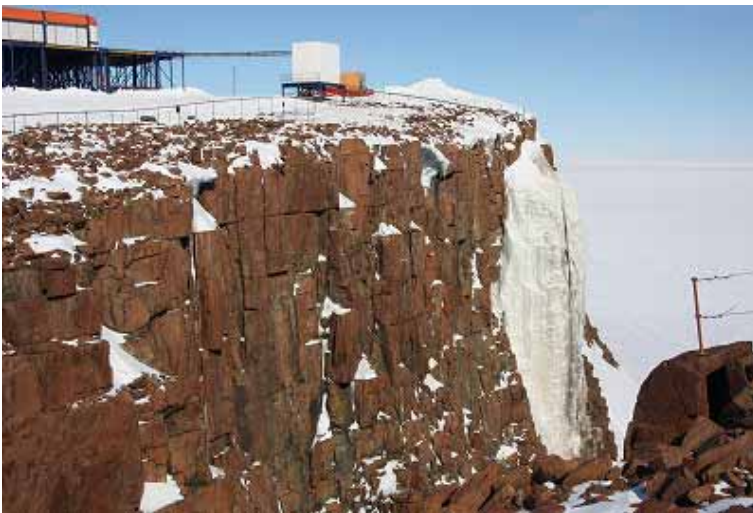
Drainage from sewage tank to the bottom of a cliff
