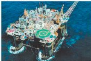
Deep water oil platform in the Gulf of Mexico. Source: shutterstock.com
