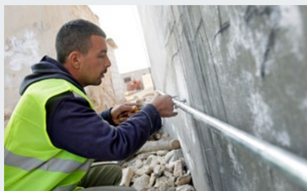
← Installment of drinking water pipes (Mafraq, Jordan)
