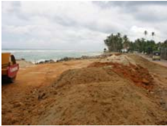
2005. 11.04 Goiyapana Bridge 建設状況 ( 1 )
