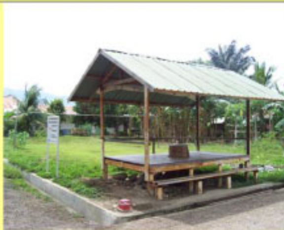
FUTURE LOCATION FOR VOCATIONAL TRAINING CENTER'S GENERAL PURPOSE BUILDING_02
