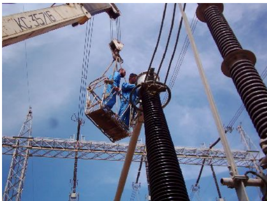
Renovation of electric substation facility
