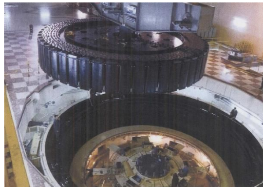
Installment of rotor for No. 2
