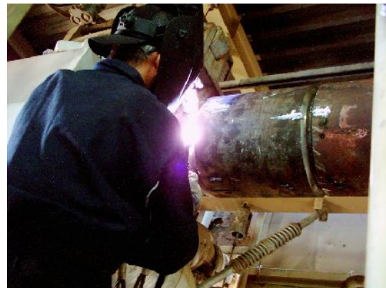
Repair of facilities within the power station
