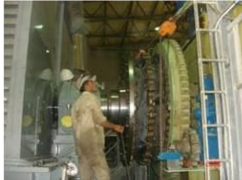
<July 2008 Installation of the diesel engine>
