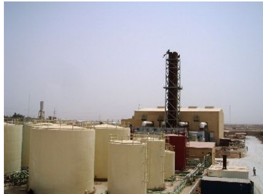
Constructed Diesel power station (May 2008)
