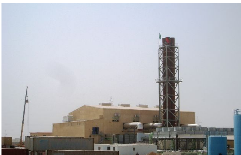
<A large-scale power station in Samawah constructed by Japan's assistance>
